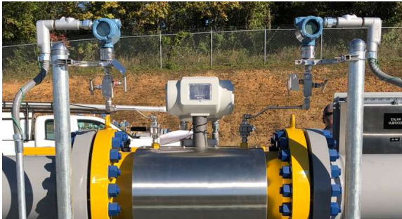
Press, Temp Transmitters
