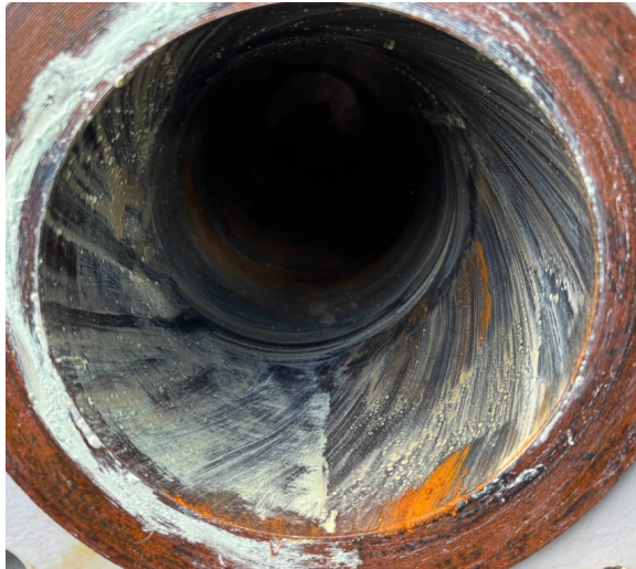
After 1 st ball hone cleaning. Hone covered by towel & degreaser used.
