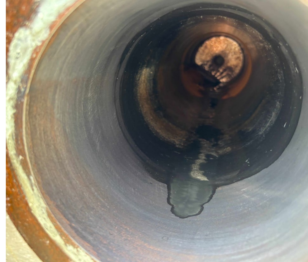
After final wiping by hand. Final condition. Some damage to coating by bare hone.
