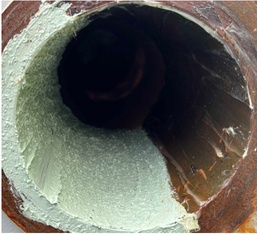
Grease & sealant added
