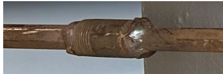
Extension that is shop fabricated square/hex bars & pipe nipples?
