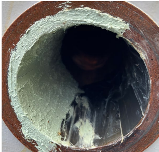
Grease & sealant added
