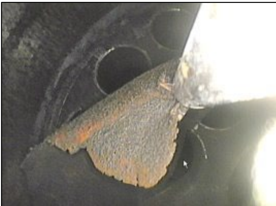
Removal of a piece of poly pig using a grabbing tool with borescope taped to the grabber
