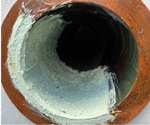
Grease & sealant added
