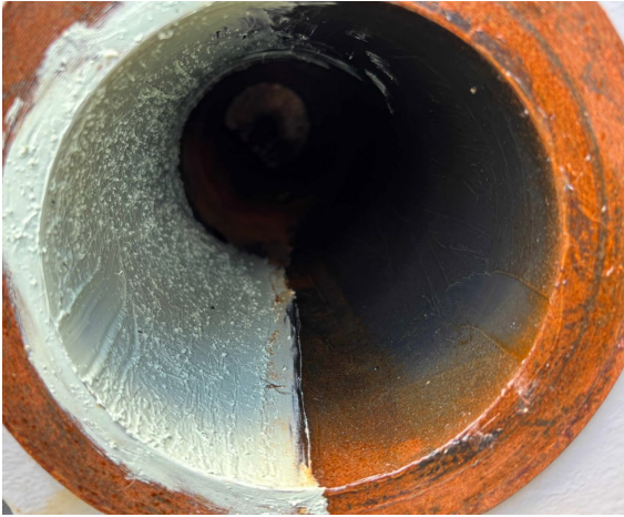
Grease & sealant added
