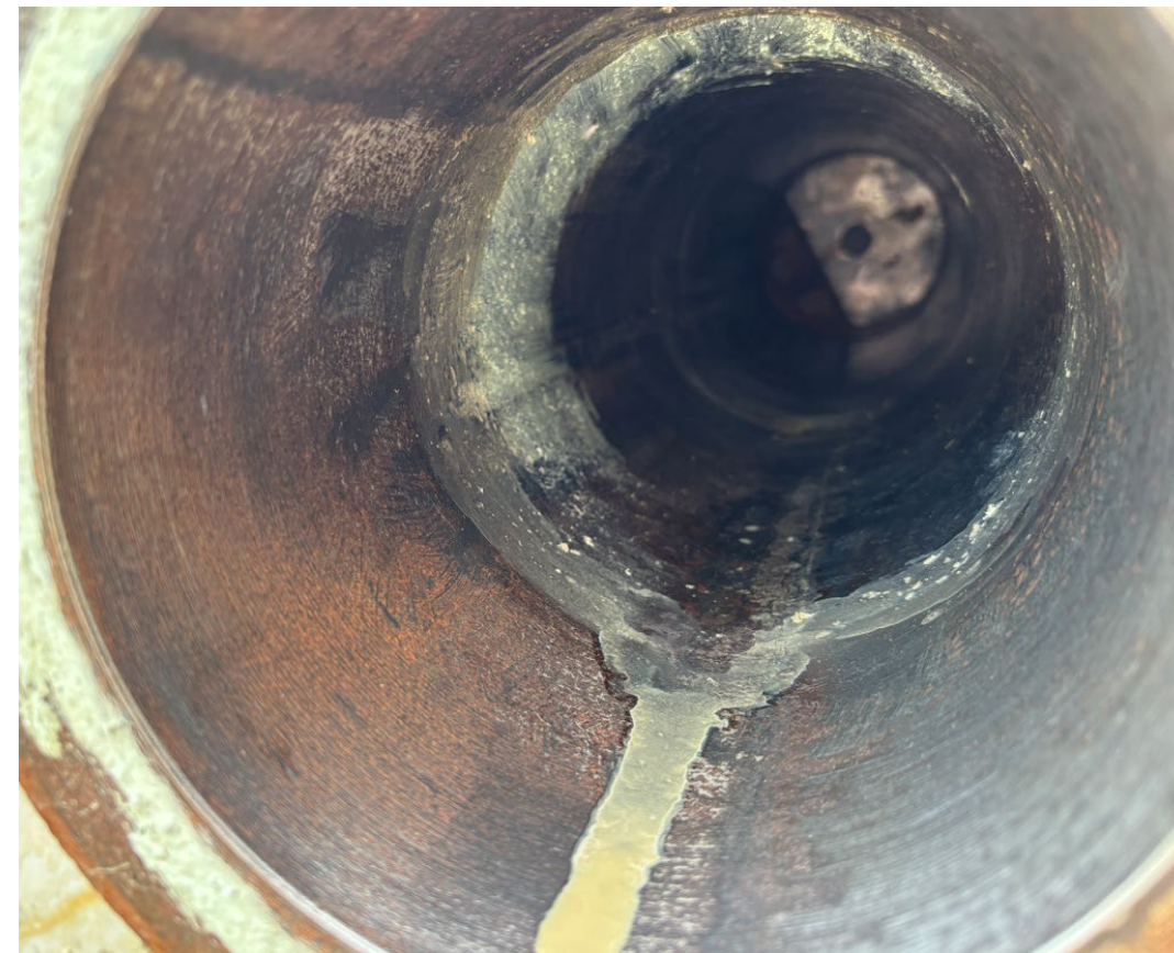
After final wiping by hand. Final condition. Damaged coating & rust showing through.
